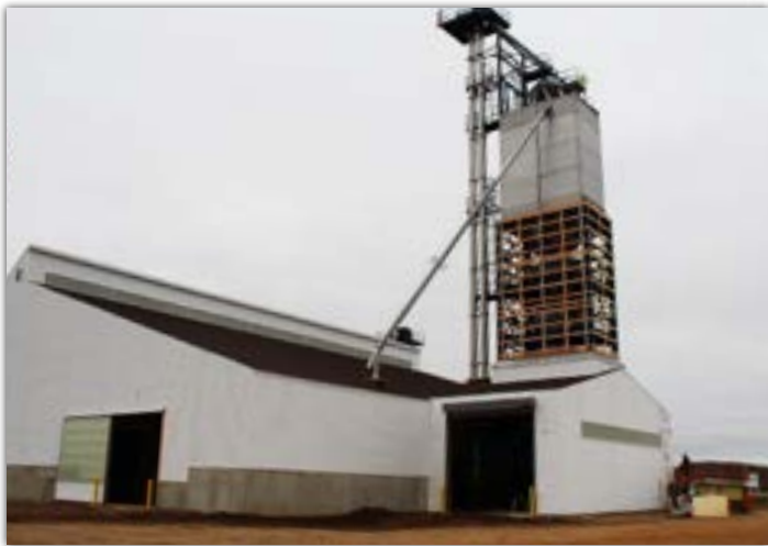
Mid-County's new fertilizer plant.
