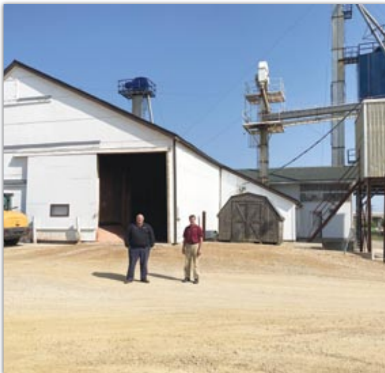
Scott Nelson and Bill Reimers stand in front of the existing dry fertilizer blending plant.
