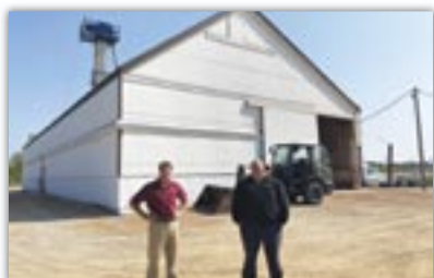
Bill Reimers and Scott Nelson stand in front of the existing dry fertilizer blending plant.
